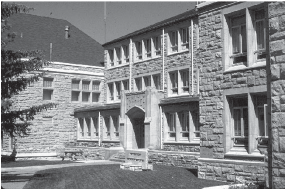
Figure 2. Geology building on the University of Wyoming Campus. The split-face stone in the wing on the left was quarried 6 miles north of Laramie around 1900. The remainder of the split-face stone is from Utah. The light colored stone around the windows is Indiana limestone, as is the cornerstone (square block right front), the steps are Lyons, Colorado, flagstone, and the trim around the low wall at the left is granite quarried 10 miles southeast of Laramie.
