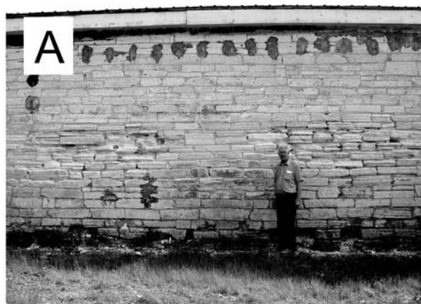
Figure 12. Charles Beebe at Wright store building, Scotia, Nebraska. A, North side of building; sawed diatomite blocks are generally tabular and of roughly uniform size, but much larger and smaller blocks appear in places. Individual blocks have weathered to different degrees. B, Weathering hollows, as much as 7 cm deep, on external surface of blocks. In an individual block, calcareous diatomite laminae also weather differentially.
