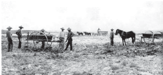
Figure 3. Harvesting of ulexite for processing into borax circa 1885, Harmony Borax Works, Death Valley, California.
