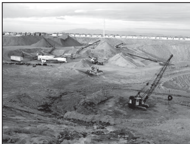
Figure 7. Las Vegas aggregate and encroaching development.
