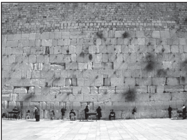
Figure 3b. Detail of the original wall.
