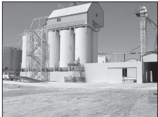
Figure 10. Lakeview processing facility.
