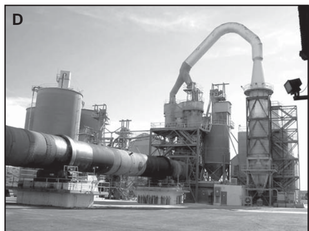
Figure 2. Views of the Nevada Cement plant: A. View of the plant from the southwest; B. View of the number 2 kiln; C. View of both kilns looking south (limestone quarry is on the ridge in the center background.); D. Number 2 kiln showing preheater.
