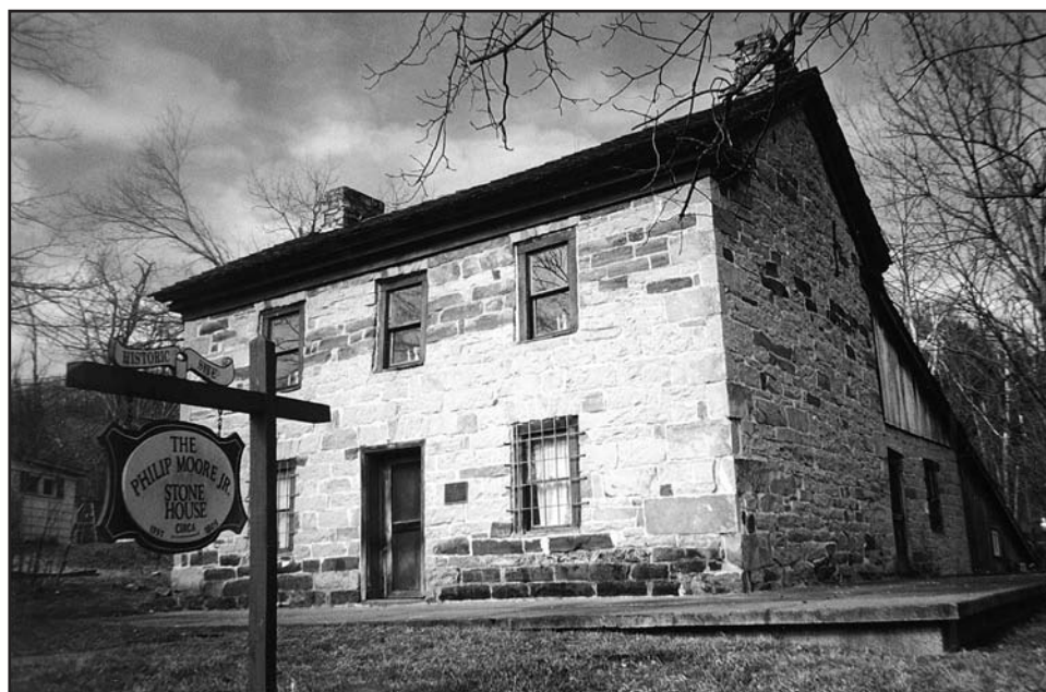
Figure 4. Front and side view of the Philip Moore Jr. home at West Portsmouth in Scioto County, Ohio. Philip was a Revolutionary War veteran and is believed to have started building the house in 1797. The house is constructed of Mississippian-age Berea Sandstone quarried from the hillside approximately 300 feet (90 m) to the south.
