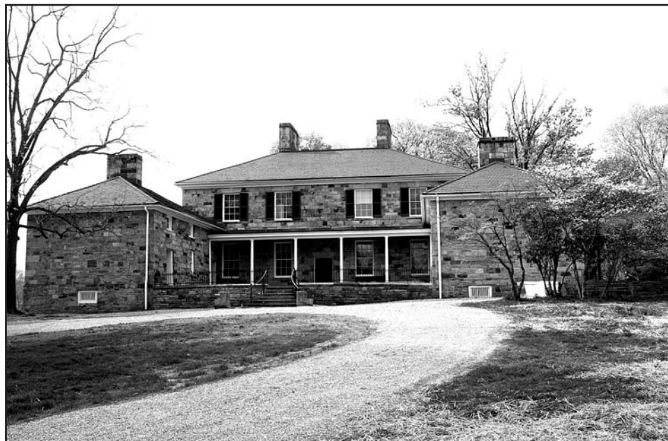
Figure 3. View of the front of Thomas Worthington's magnificent estate, Adena , constructed in 1807 overlooking the Scioto River Valley and Chillicothe in Ross County, Ohio. The Mississippian-age Berea Sandstone used to build the estate was quarried onsite.
