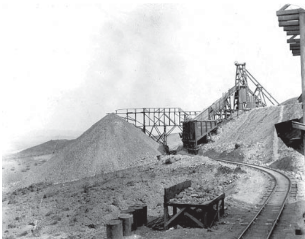
Figure 4. High Point Shaft 1902, Old Borate, Calico Mountains, California.
