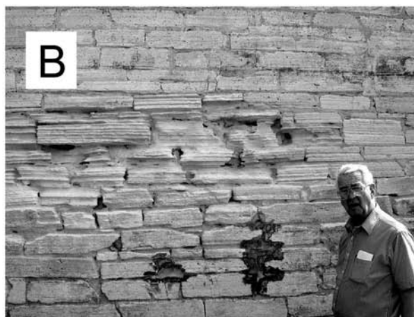
Figure 12. Charles Beebe at Wright store building, Scotia, Nebraska. A, North side of building; sawed diatomite blocks are generally tabular and of roughly uniform size, but much larger and smaller blocks appear in places. Individual blocks have weathered to different degrees. B, Weathering hollows, as much as 7 cm deep, on external surface of blocks. In an individual block, calcareous diatomite laminae also weather differentially.
