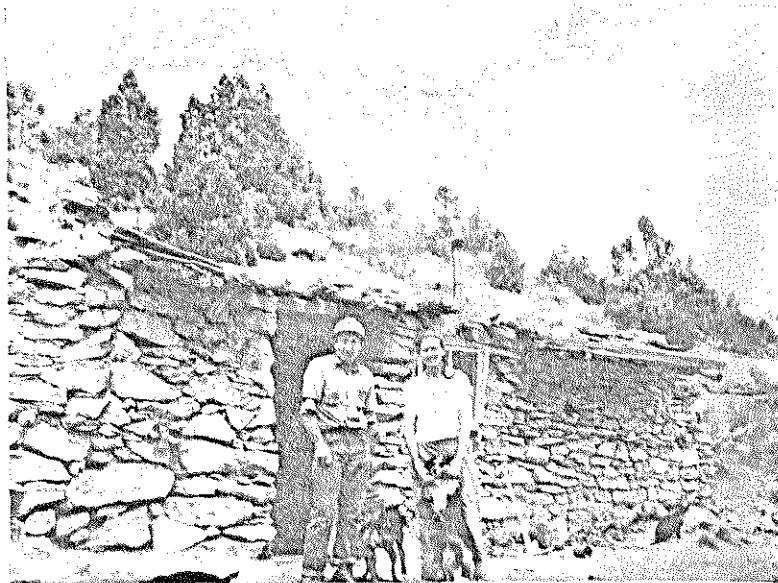
(2) Native stone was a common early day building material. Upper. Joe Clifford and one of the stone cabins. This is one of the original buildings of the landmark, the construction of which began about 1862.
