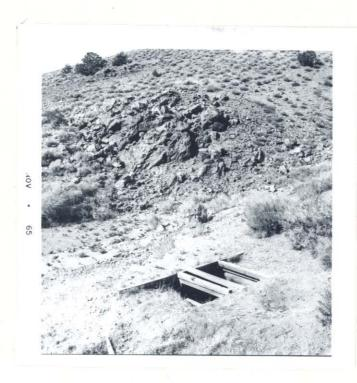
Photo No. 1. View, looking N. 60° W., showing collar to 88-foot shaft in foreground and outcrop of mineralized structure in center background.
