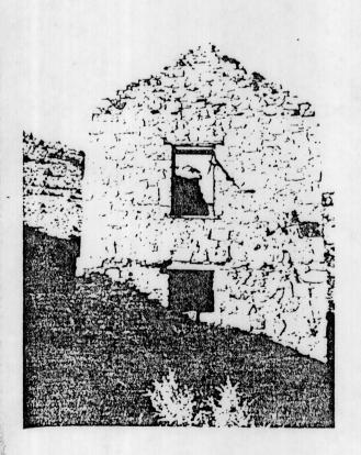
One 2-story angular rock structure measured 50'-6" x 17'-6" x 20 feet high. The 20-inch-thick walls are mortared; the interior is plastered. The ground floor is concrete, and the second floor is of wood construction. The medium-rise gable no longer supports a roof; some loose rock was observed where the roof would have made contact. The long axis trends north-south, and the east-facing elevation has 50% fenestration. The west elevation
