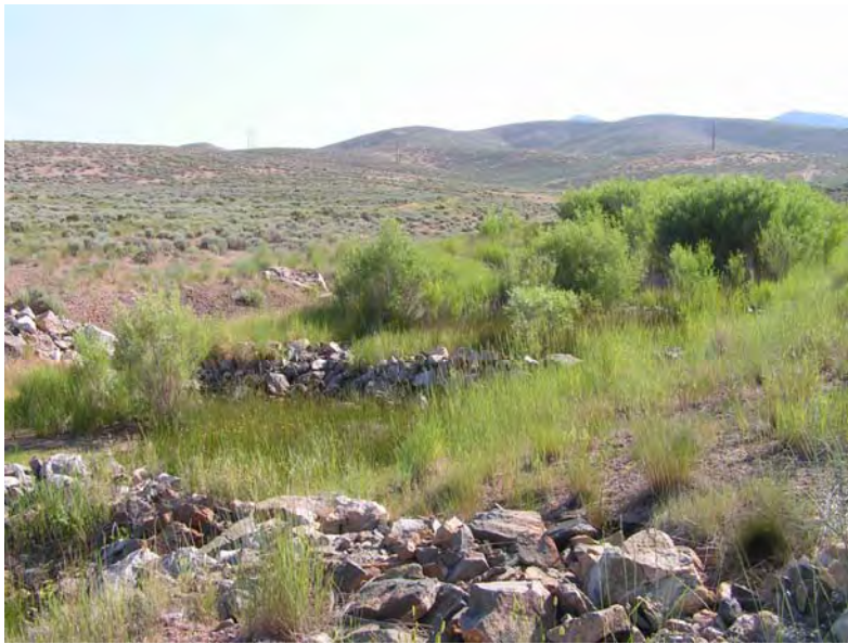
Photo No. 1: Relocation of tributary to Bell Creek northwest of Carlin, Nevada, illustrates conceptual design for construction of engineered stream channel in the Emigrant drainage. Relocated channel includes sinuous meandering channel cobble bed, rock weirs, and riparian vegetation including willows, sedges, and rushes.
