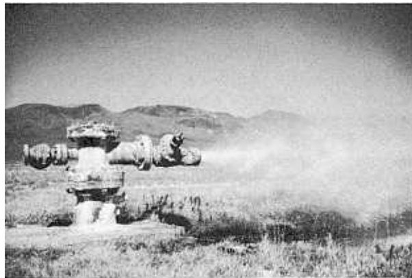
Steam well at Wabuska Hot Springs, Lyon County.
